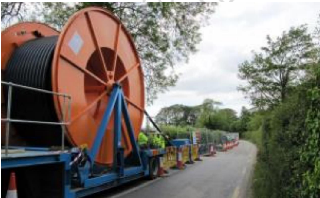
Figure 4.13: Cable Drum at Joint-bay location
