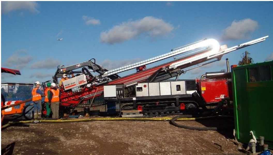
Figure 4.7: Photo of Typical maxi-rig HDD Drill Rig
